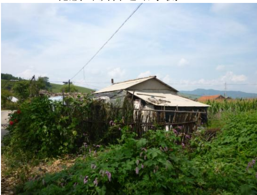
驼腰岭镇转运站北侧
